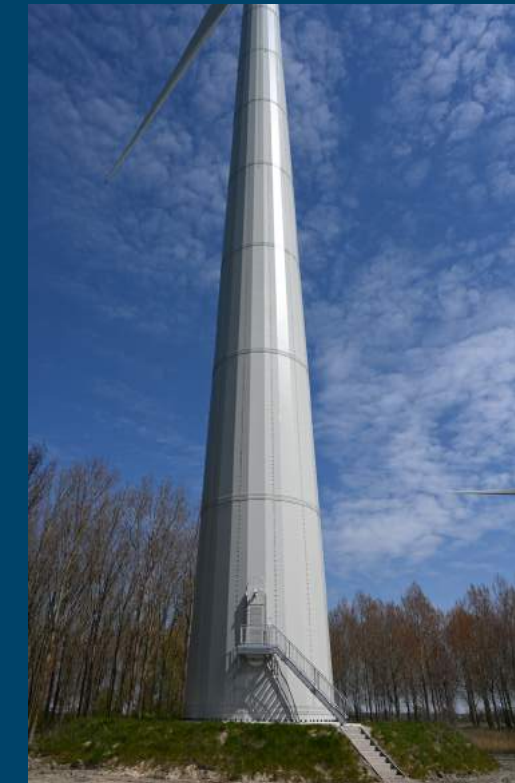
Windpark Westerse Polder
