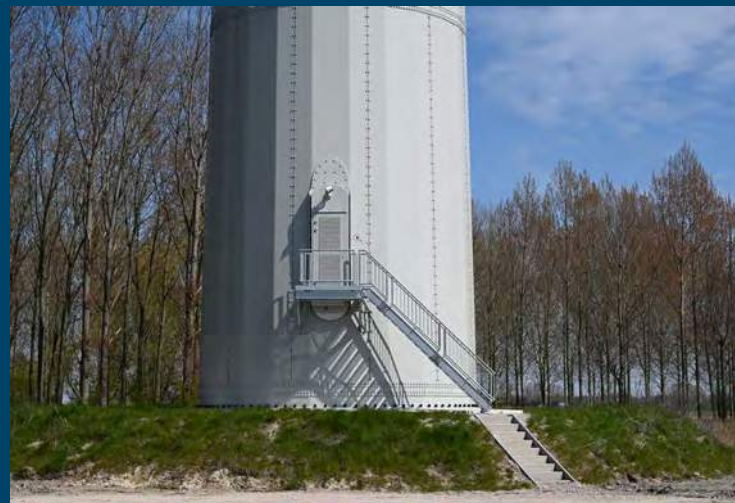
Windpark Westerse polder
