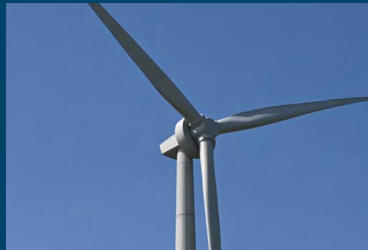
Windpark Westerse polder
